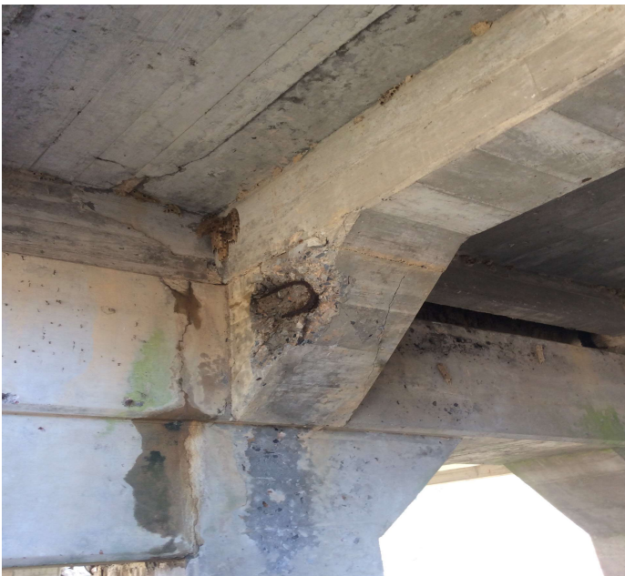
PHOTO 1 Description Span 3 Girder 4 @ Bent 3: Exposed rebar
