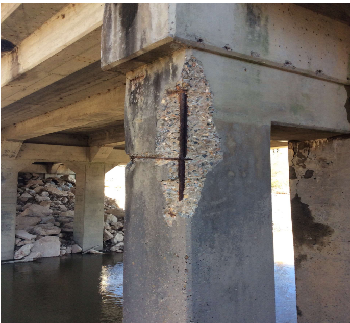
PHOTO 1 Description Bent 3 - Column 5: Exposed rebar
