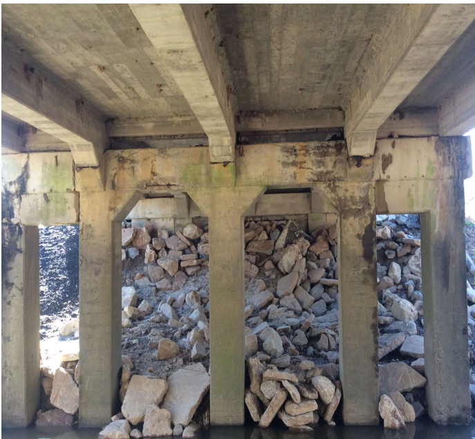
PHOTO 1 Description Cap - Bent 3: Cracking/exposed rebar
