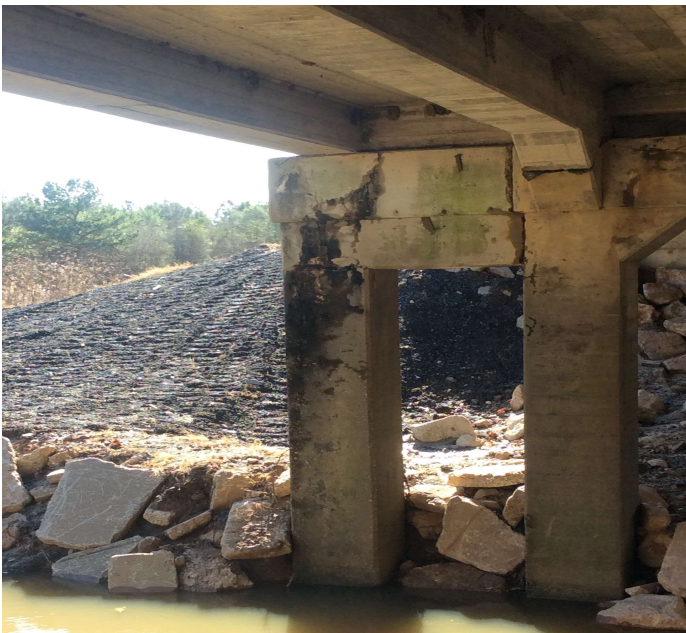
PHOTO 1 Description Bent 3 - Column 1: Steel exposed
